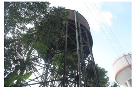
Raj Rajeshewari Water Works
