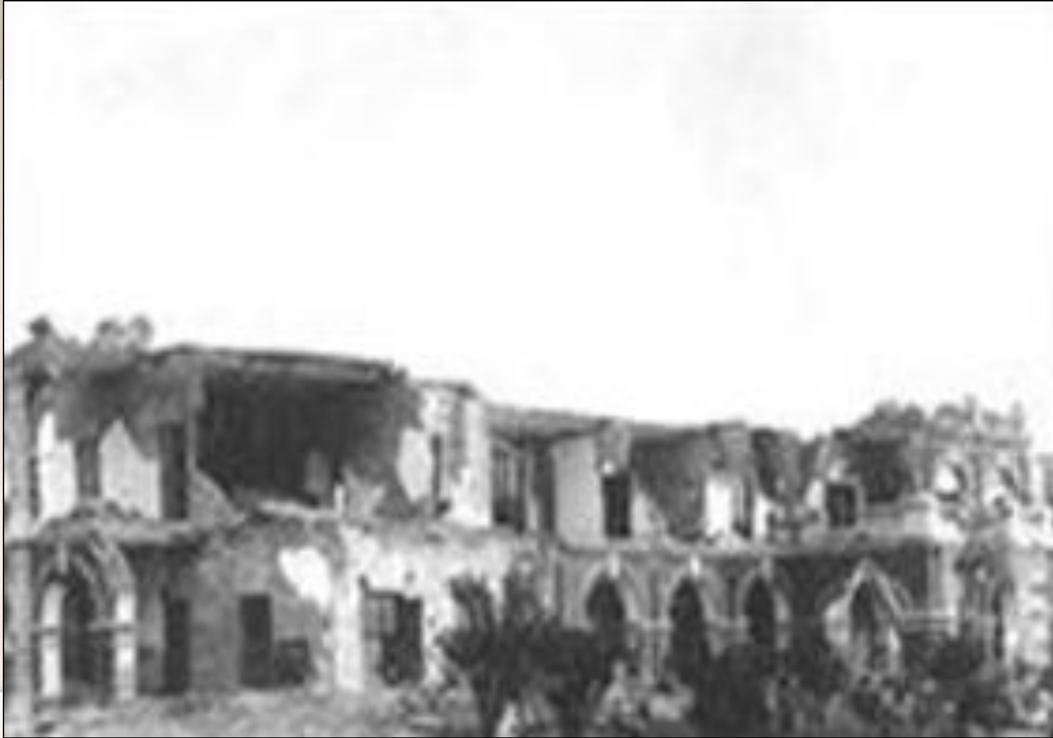
Damaged Court Building of Mymensingh due to earthquake in 1897 with 8.7 Mw
